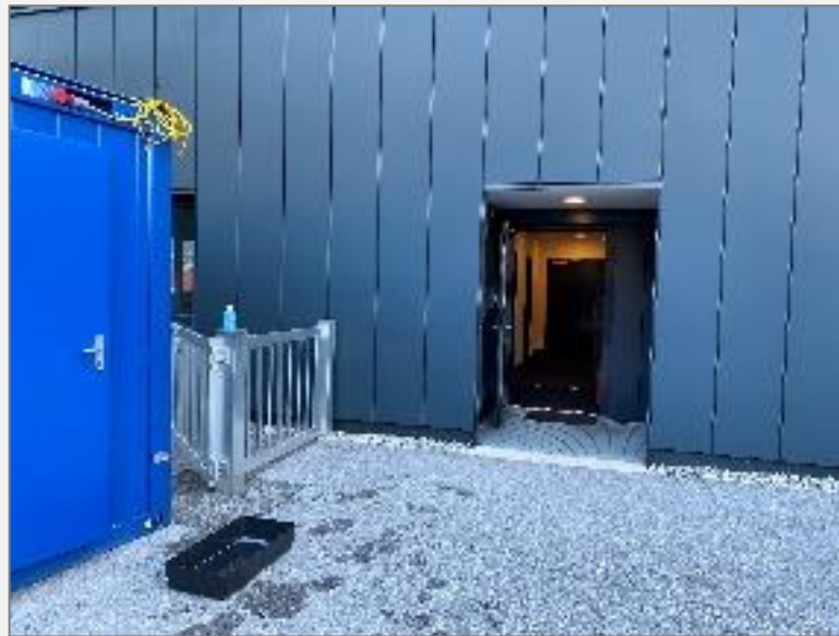
Disinfections bath area
